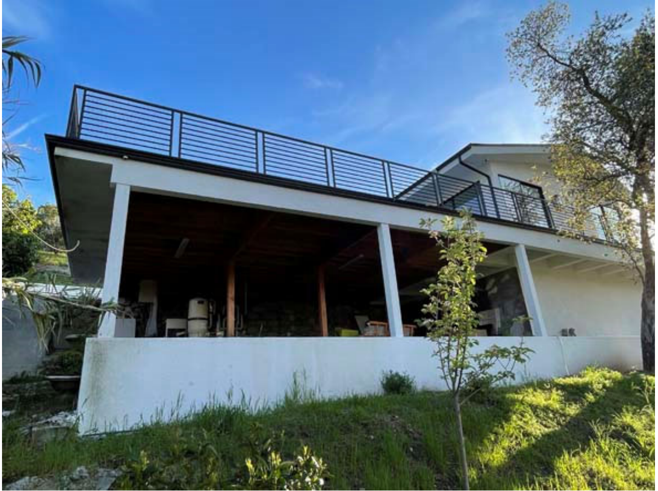
Figure 28: Looking southwest at the rear deck.
