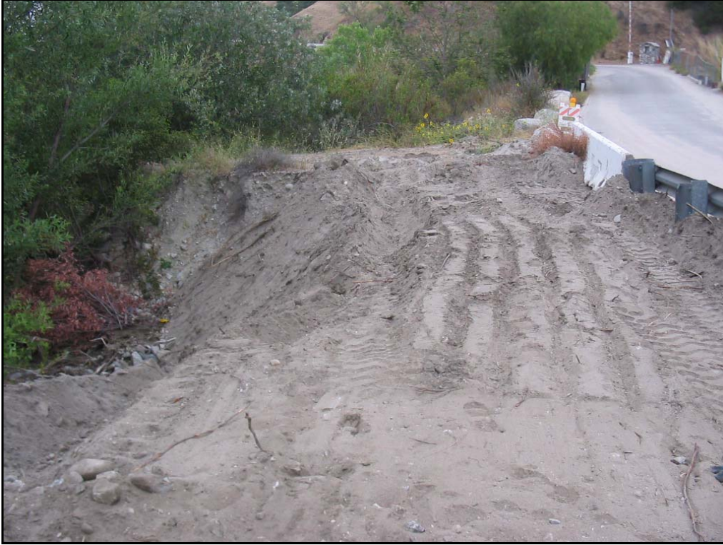
Figure 5. Post-construction, with water no longer flowing over Oro Vista Avenue.
