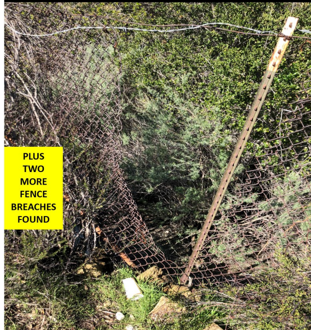
FEB 16, 2019 8AM – PRIOR FENCE BREACH + 2 NEW
