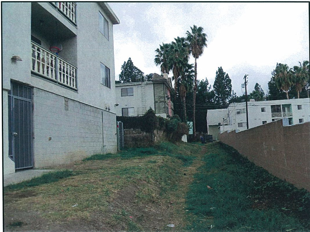
SOUTH VIEW AT REAR OF EXISTING APARTMENTS
