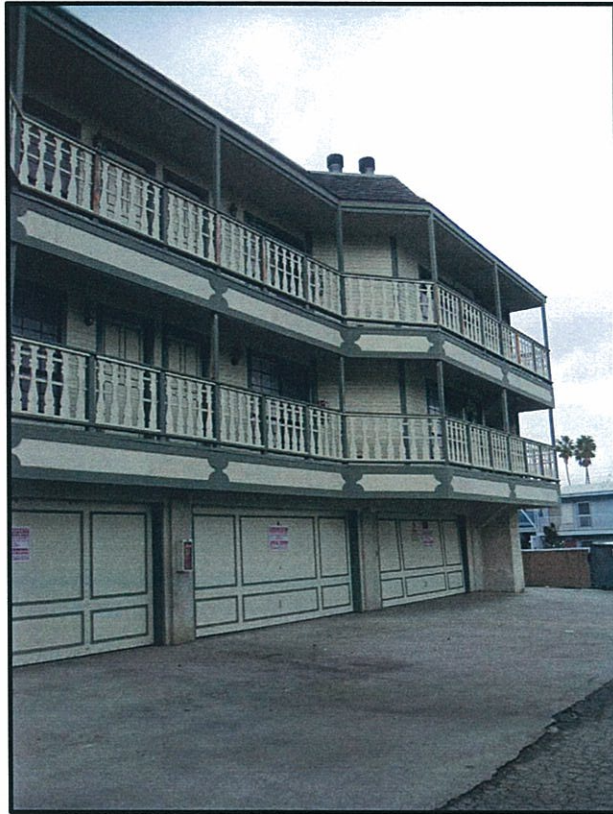
WEST VIEW AT EXISTING APARTMENTS
