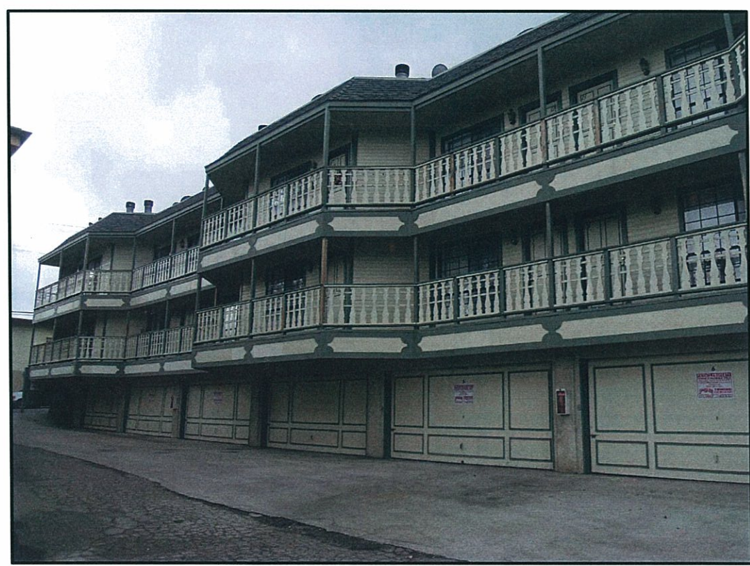
EAST VIEW AT EXISTING APARTMENTS
