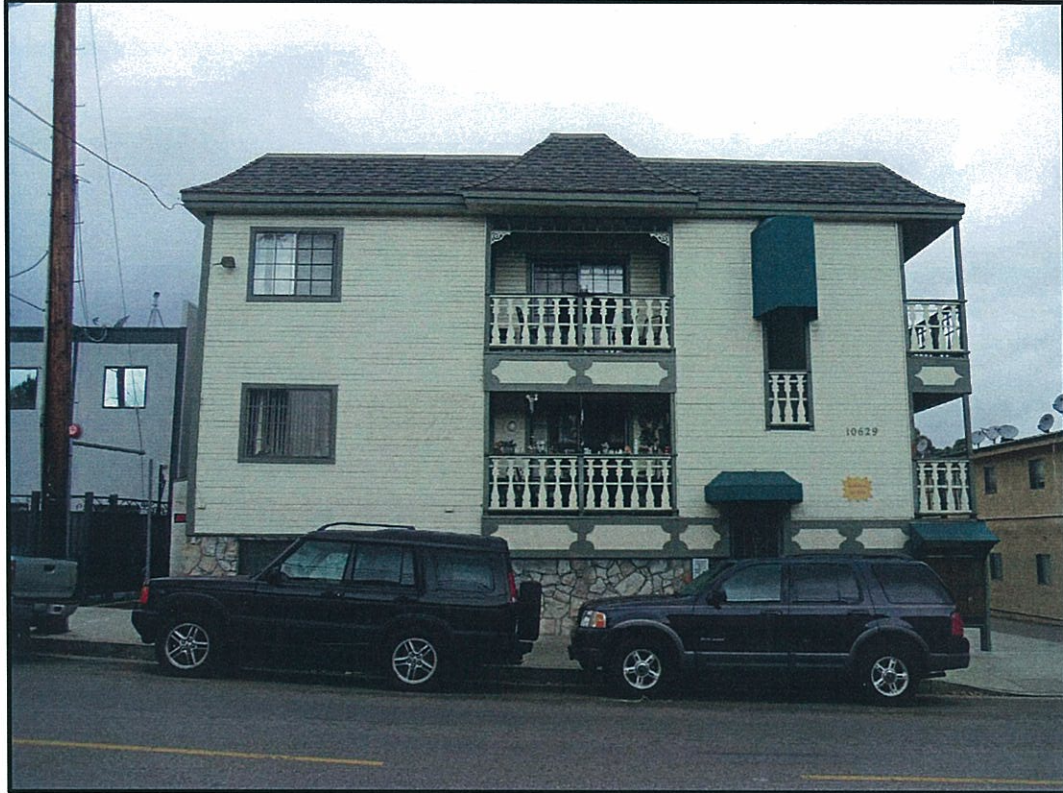
LOT FRONTAGE WEST VIEW AT EXISTING ENTRANCE TO EXISTING APARTMENTS
