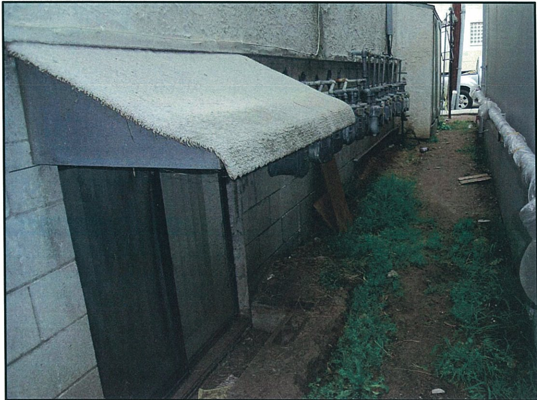
EAST VIEW AT SIDE YARD OF EXISTING APARTMENTS
