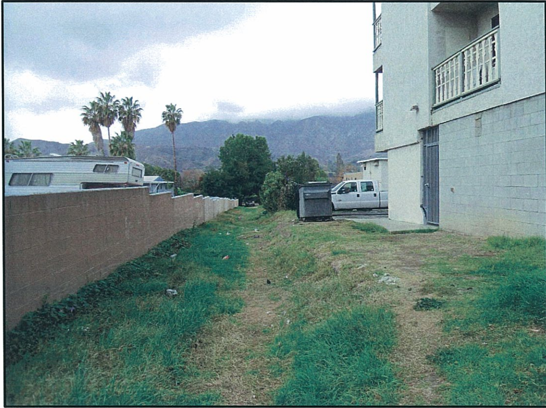
NORTH VIEW AT REAR OF EXISTING APARTMENTS
