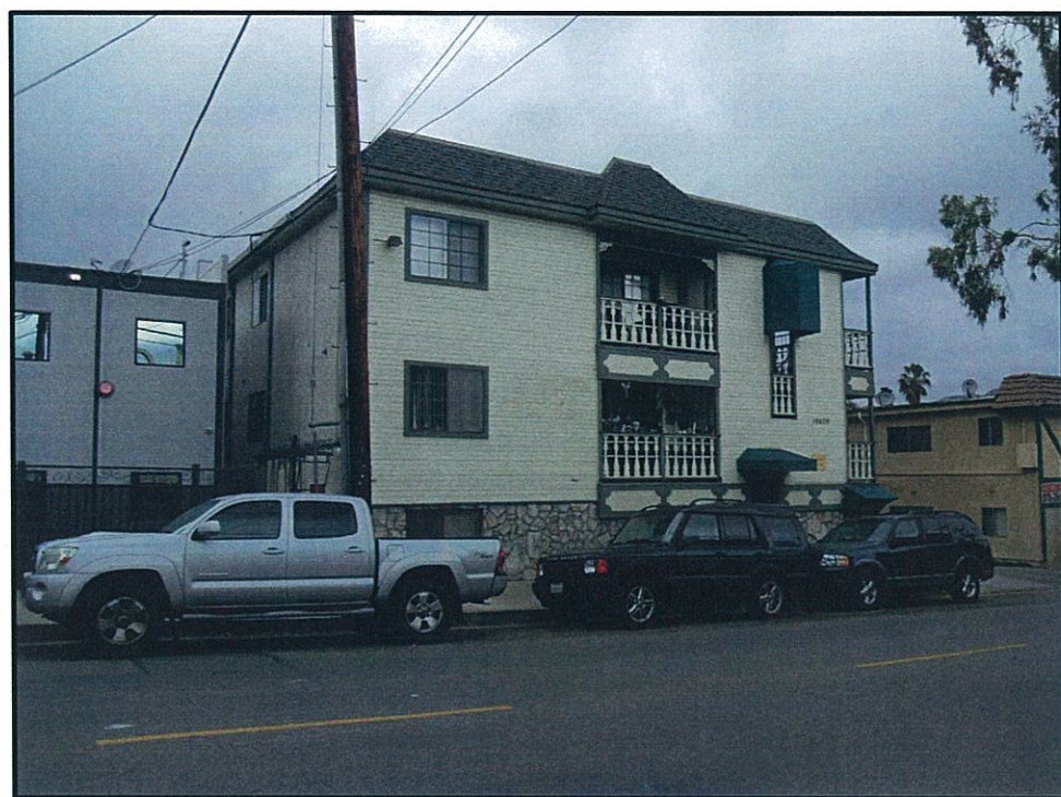
LOTS MAIN FRONT STREET NORTHWEST VIEW AT EXISTING APARTMENTS
