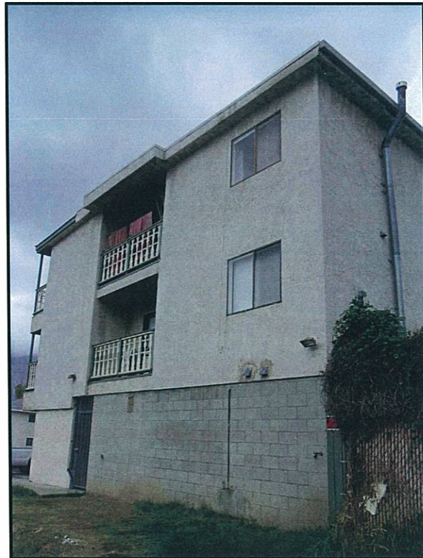
SOUTHEAST VIEW AT REAR OF EXISTING APARTMENTS
