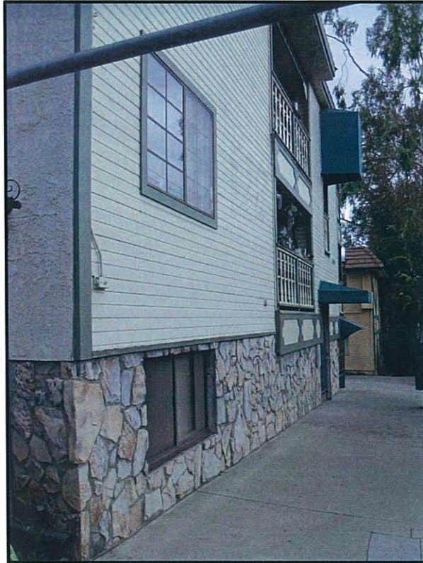
NORTH VIEW OF MAIN FRONT ENTRANCE AT EXISTING APARTMENTS
